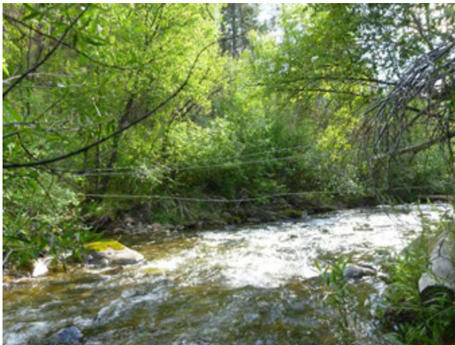
Fig. 32: Drift fence crossing Castle Creek, with lowest wire broken. 44.822167° N, 114.497108° W.
