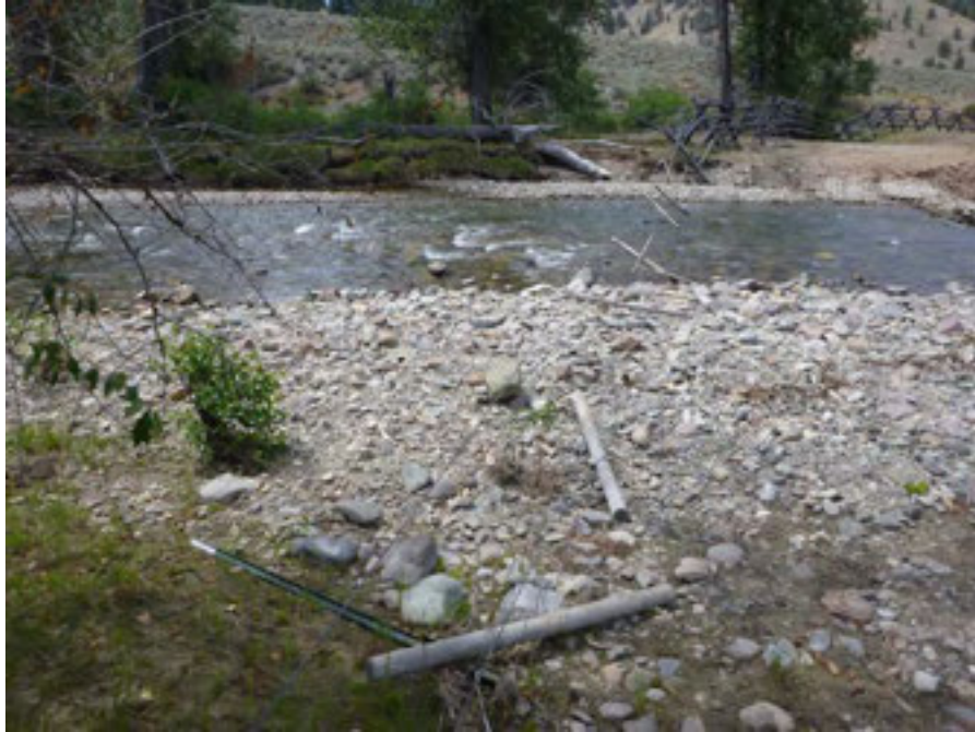
Fig. 2: Fence on right bank of upstream side of West Fork ford lying on ground. 44.829775° N, 114.496642° W.
