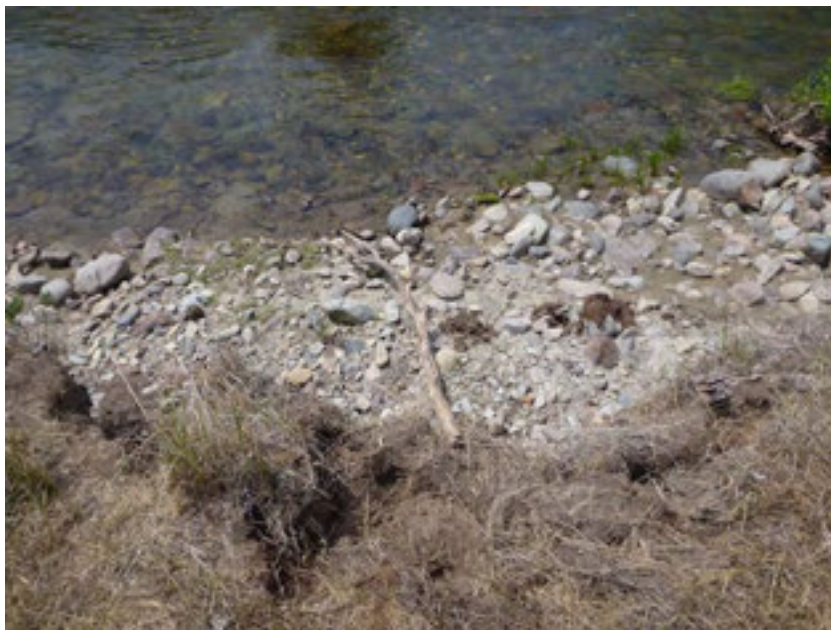
Fig. 8: Slumping right bank of Camas Creek, upstream of West Fork ford; fresh cow waste visible on gravel. 44.825131° N, 114.500042° W
