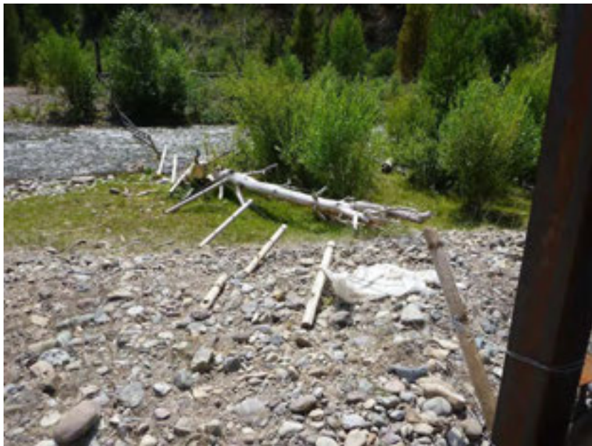
Fig. 23. Collapsed fence on right bank, upstream end of exclosure. 44.822206°N, 114.497031° W.
