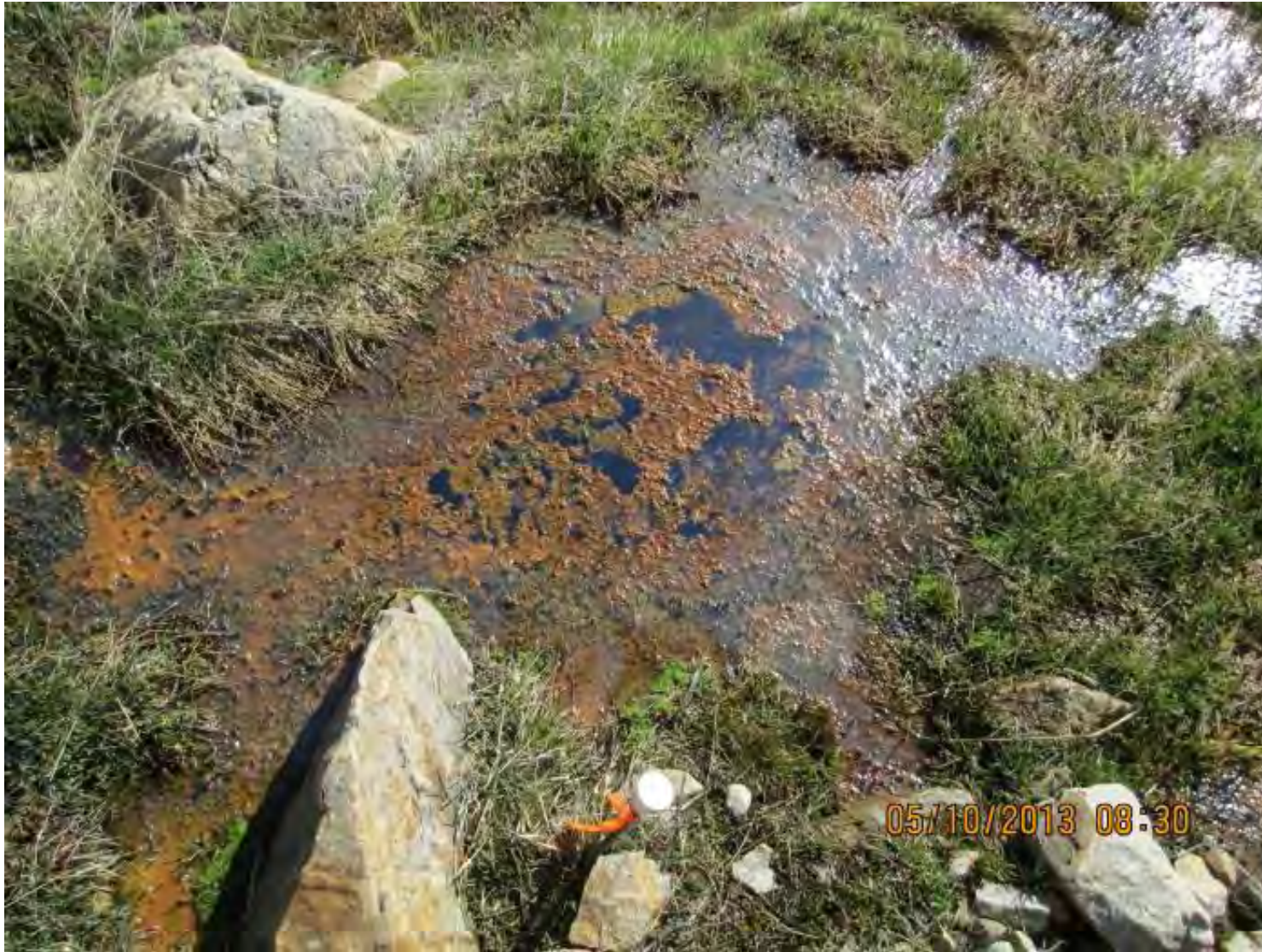
Figure 4F. Photo of the Middle Keyway Dam seep (YP-S-7) from the Surface Water Quality Baseline Study, Appendix G, May 2013 Site Photos, page 15. Photo caption reads, "YP-S-7, Middle Keyway Dam seep. Close-up looking east and downstream at seep source emerging from base of dam. May 2013."
