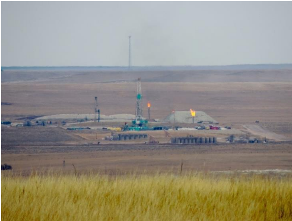
Visible flaring and air-quality impacts from oil and gas infrastructure.
