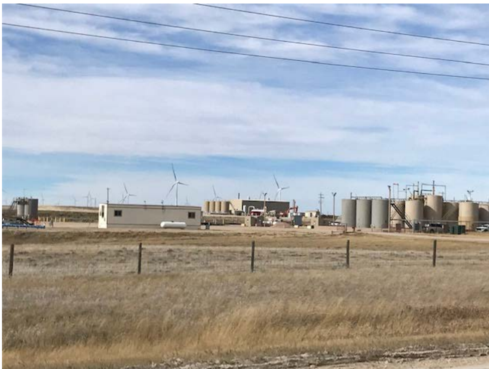
Well pad and infrastructure in Project Area. Photo: Maria Katherman
