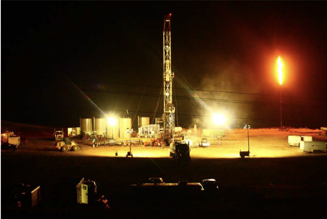
Well pad, workover rig, and flare at night. Photo: SkyTruth
