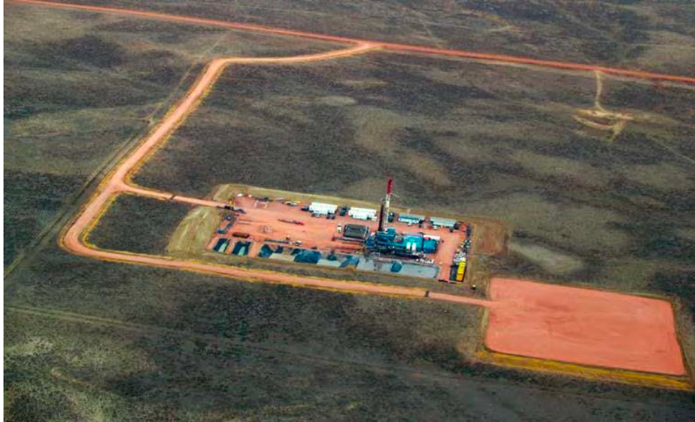
Two well pads in Converse County. Photo: Erik Molvar/WWP
