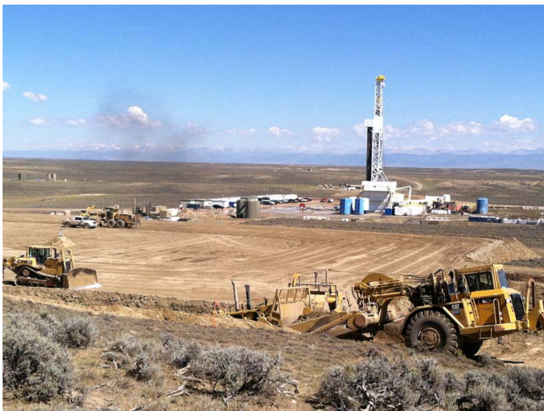
Bulldozing oil and gas well pad in Wyoming. Photo: WildEarth Guardians
