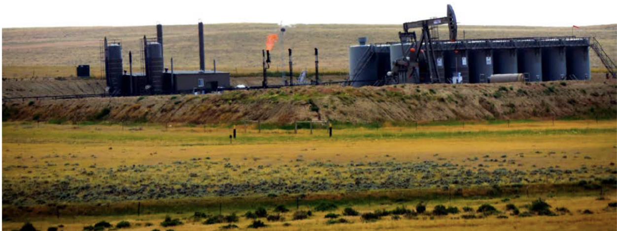
Producing well pad and flare in Powder River Basin. Photo: WildEarth Guardians
