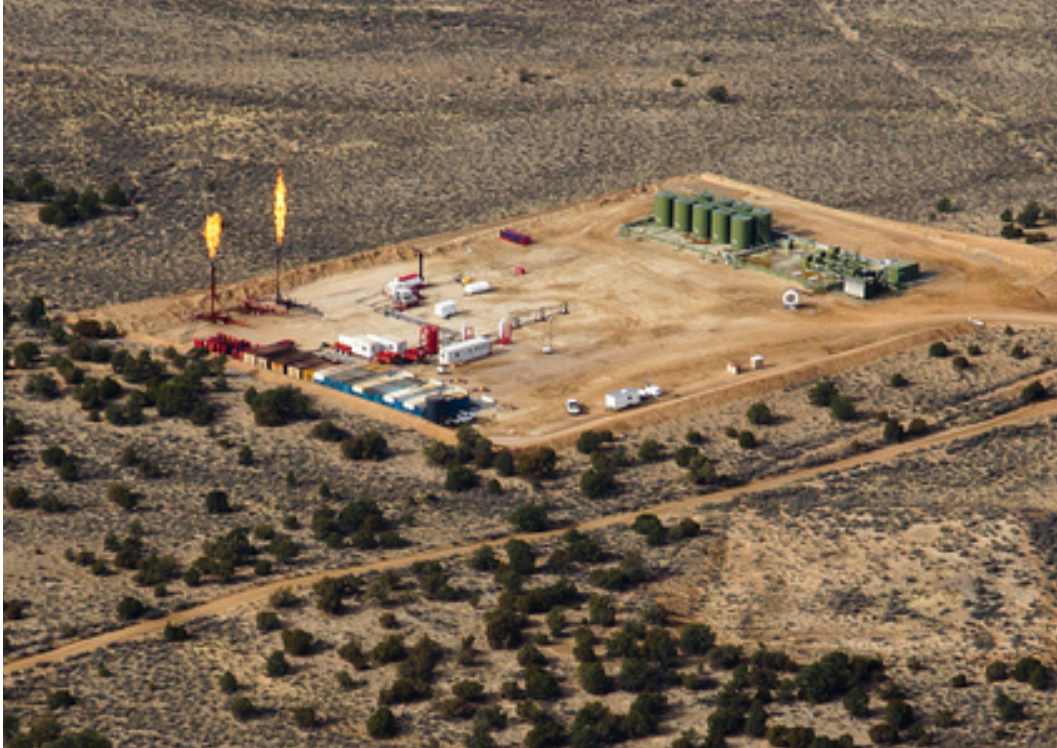
Flaring and well pad. Photo: EcoFlight
